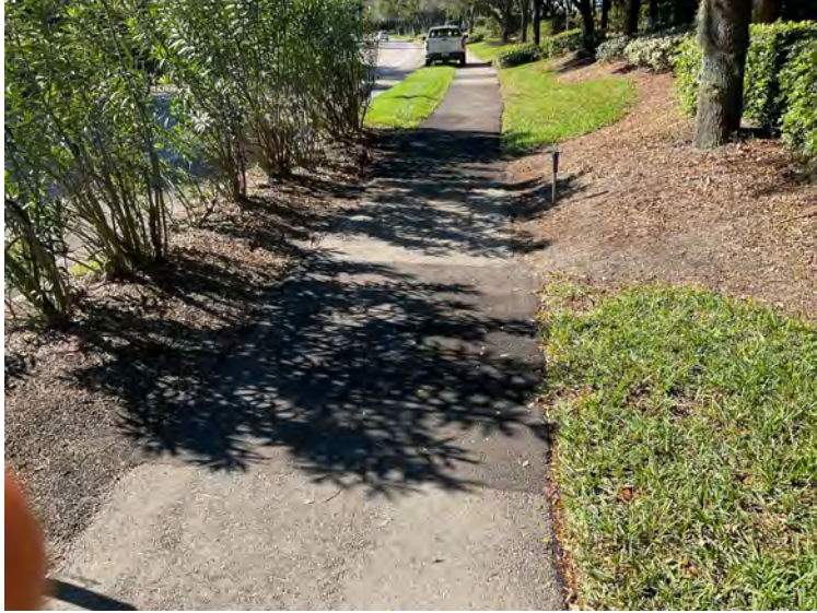
Area 5 – Light Post 23: 90' of Root Barrier
