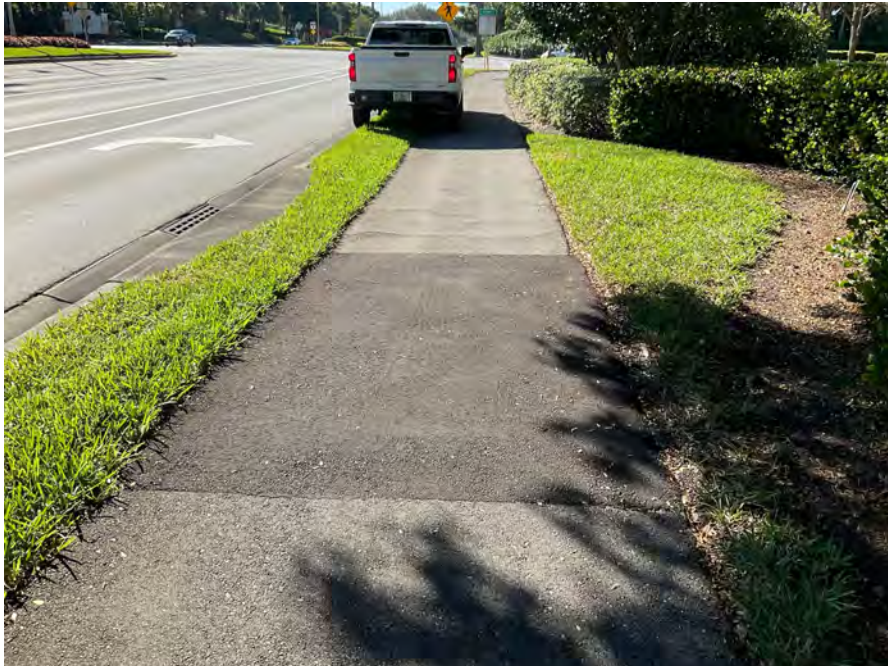
Area 6 – Light Post 12: 15' of Root Barrier
